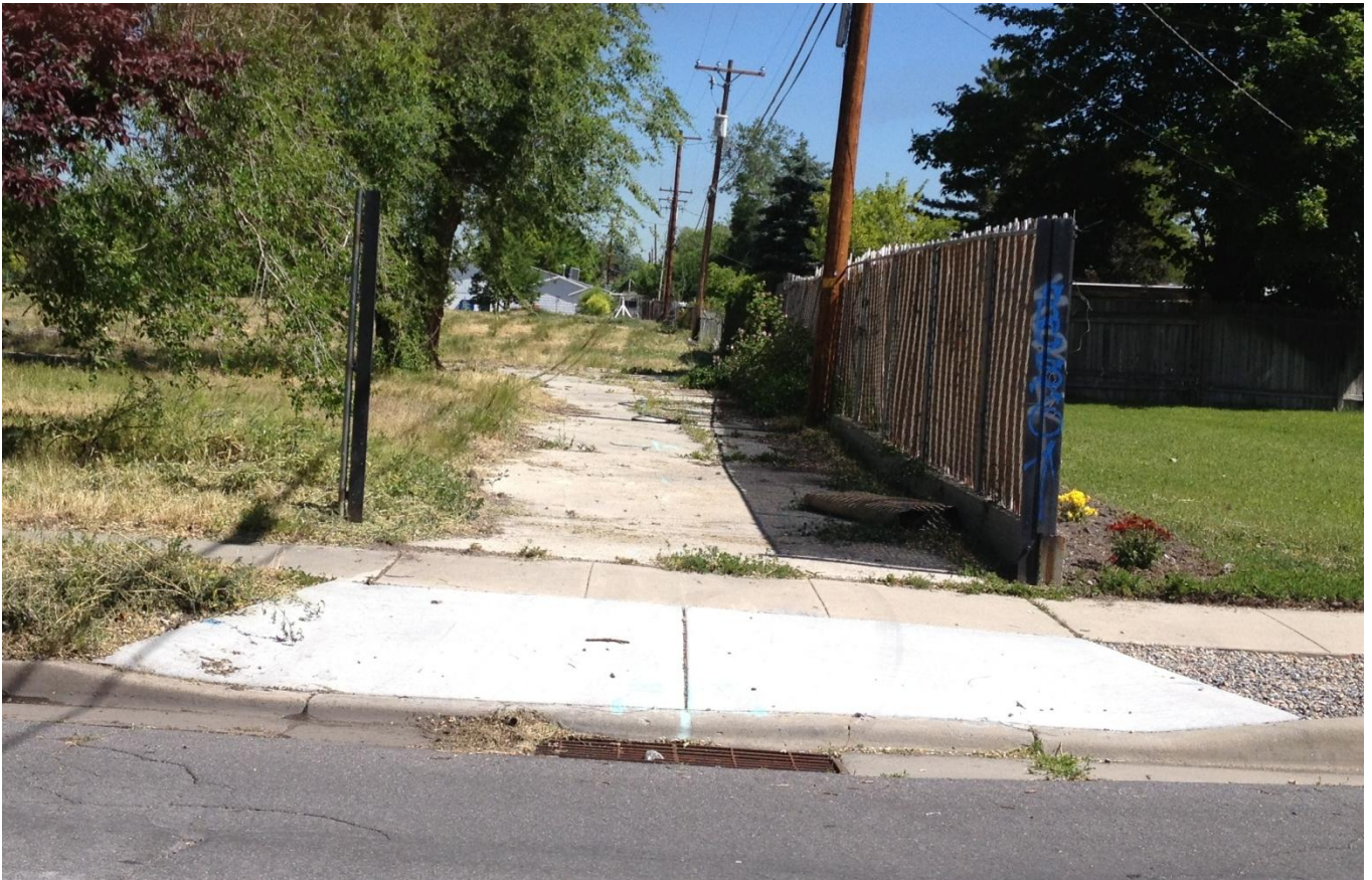
View of alley from south entrance (looking north from 1400 S)
